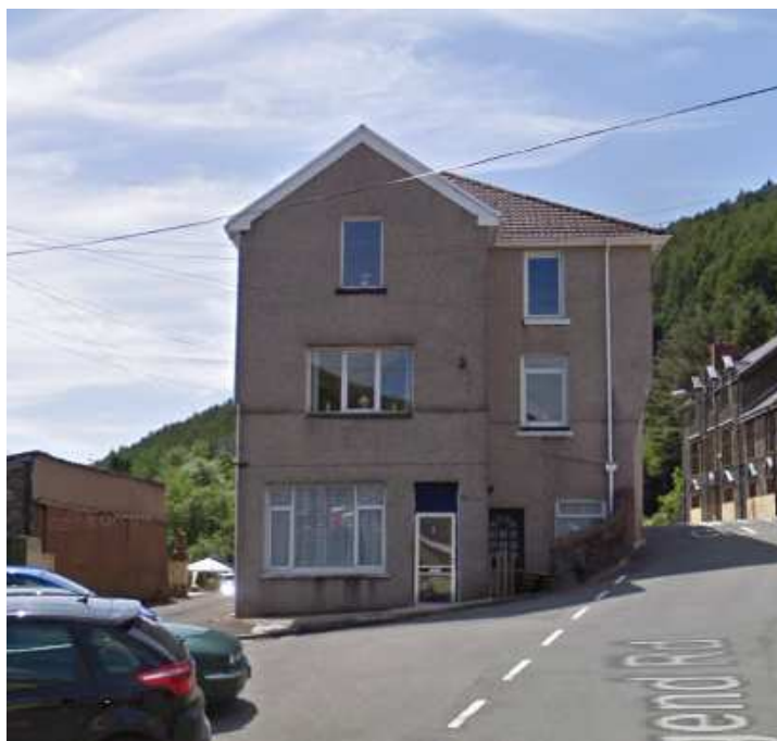
Figure 3 – Front elevation of 1/1A Chapel Street
